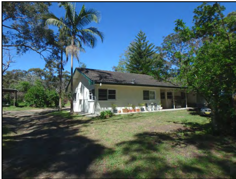
Figure 7: Residential dwelling and associated vehicle access (driveway) at the front (north end) of the property. View south west.
