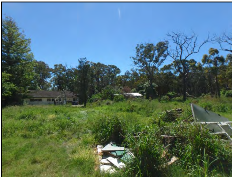
Figure 9: Thick vegetation and rubbish at the rear of the residential dwelling. View north.
